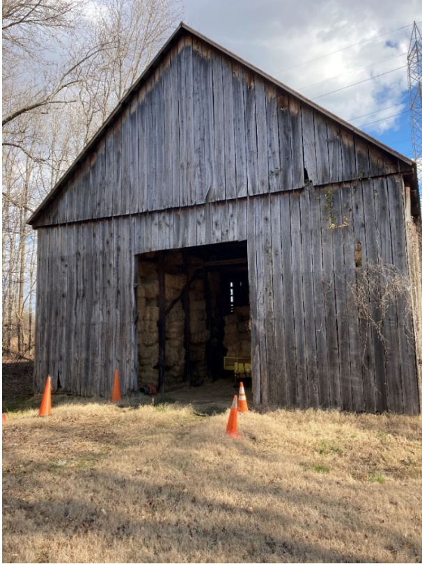
Existing Wooden Barn
