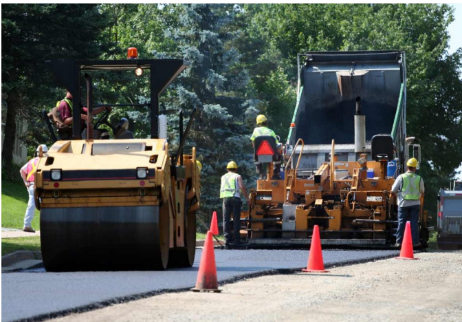
3. Typical asphalt pavement installation operation.
