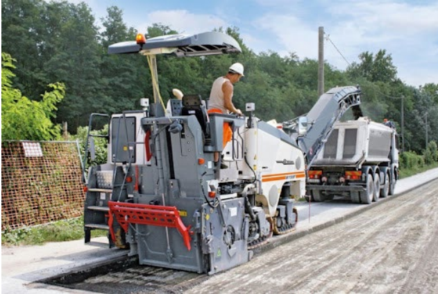
1. Typical asphalt pavement milling operation.
