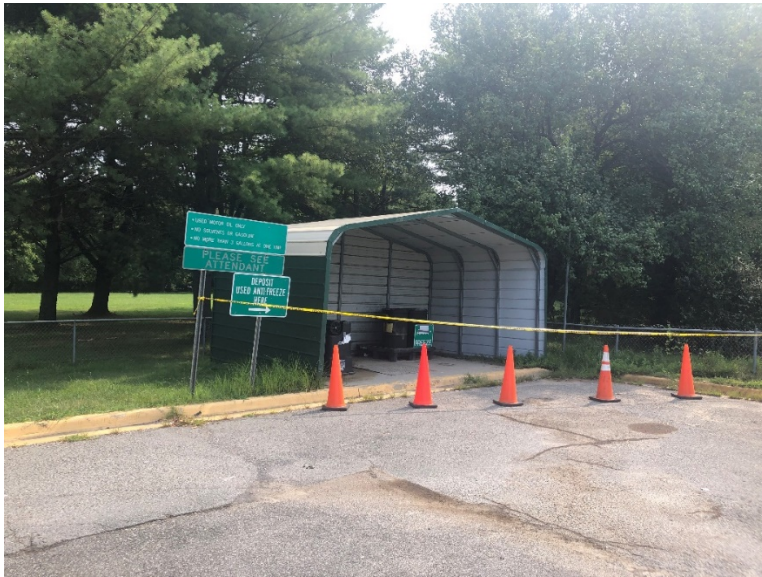
Figure 1: Existing Convenience Center at BSRSL
