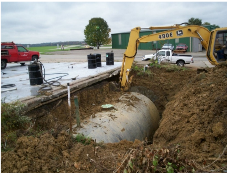
Figure 2: Typical UST Removal (stock image)
