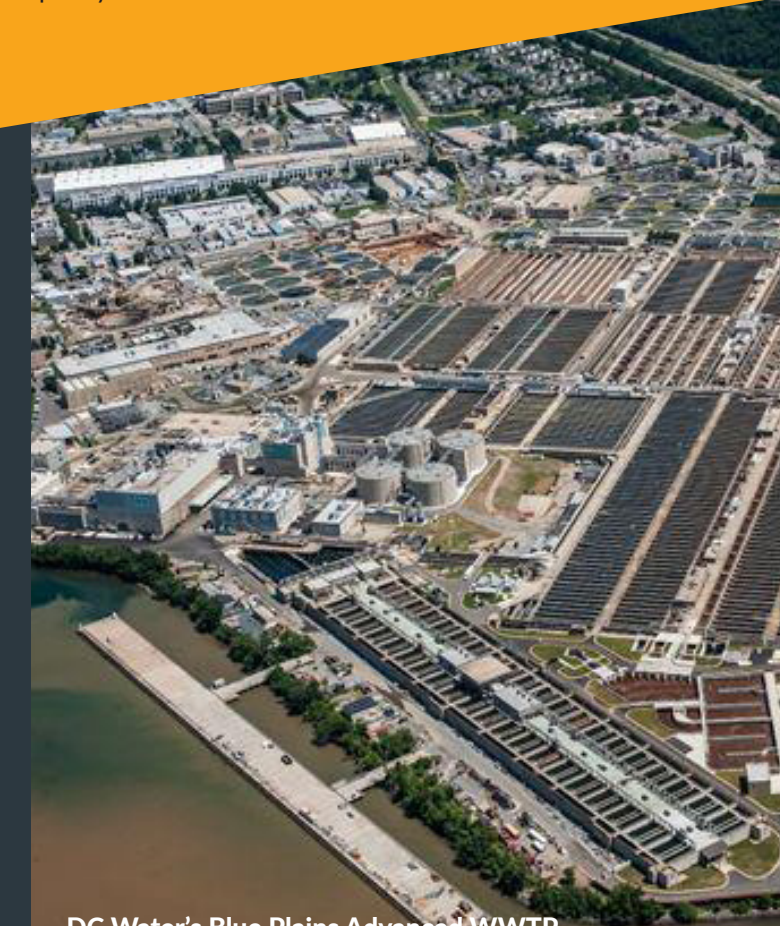
DC Water's Blue Plains Advanced WWTP
