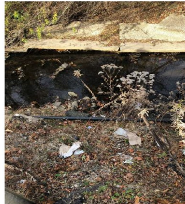
D7 MD 108 at Lark Brown Rd, Howard County, 7 Dec 2021, HO319 Stream out of flume and eroding slope, debris blockage, sign foundation exposed, unknown utility exposed
