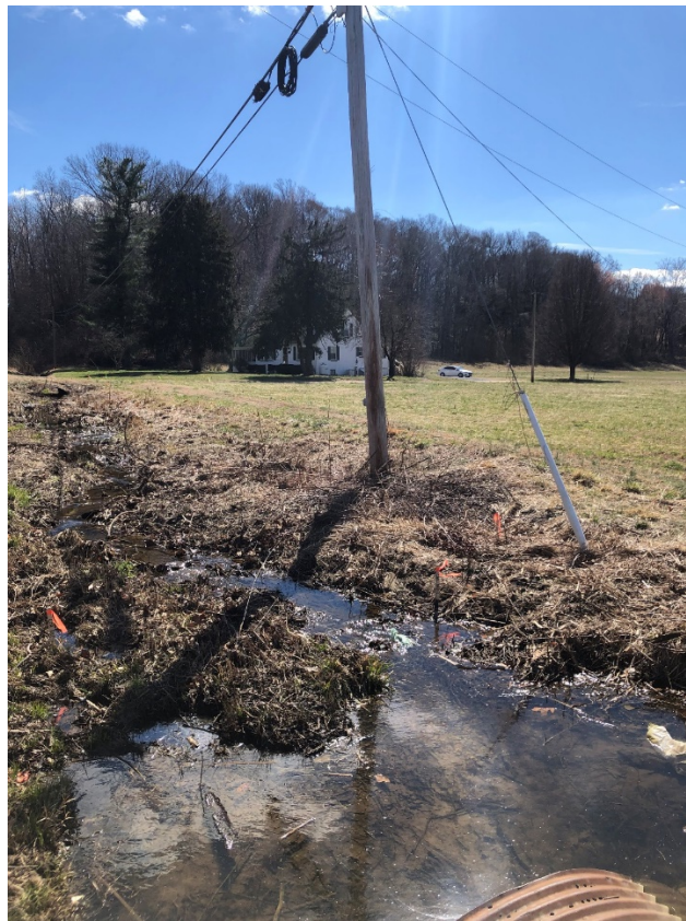
Image 3: Filled drainage swale, to be excavated, MD 234 Budd's Creek
