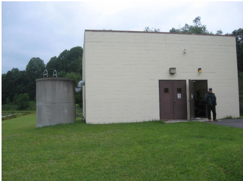
Wastewater Treatment Plant Building
