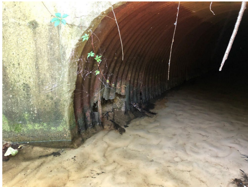
Picture 2: MD 100 Infiltration Basin – Failed Corrugated Metal Pipe and Accumulated Sediment
