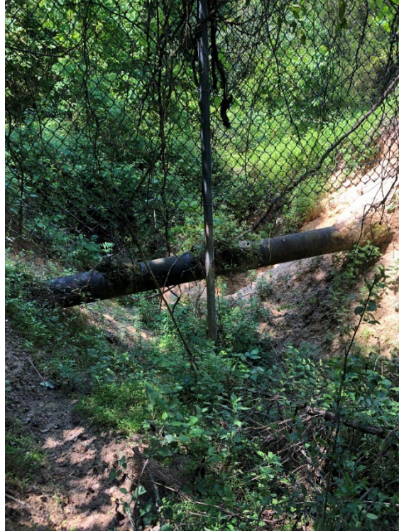
Picture 2: MD 100 Infiltration Basin – Failed Corrugated Metal Pipe and Accumulated Sediment
