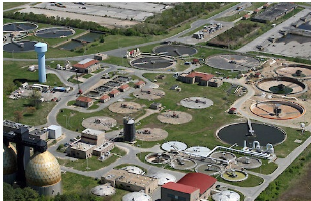
Back River WWTP – Aerial View of Digestion System
