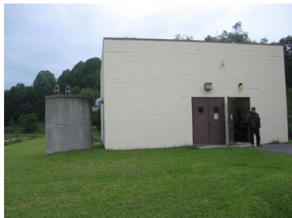
Wastewater Treatment Plant Building
