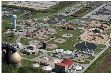
Back River WWTP – Aerial View of Digestion System
