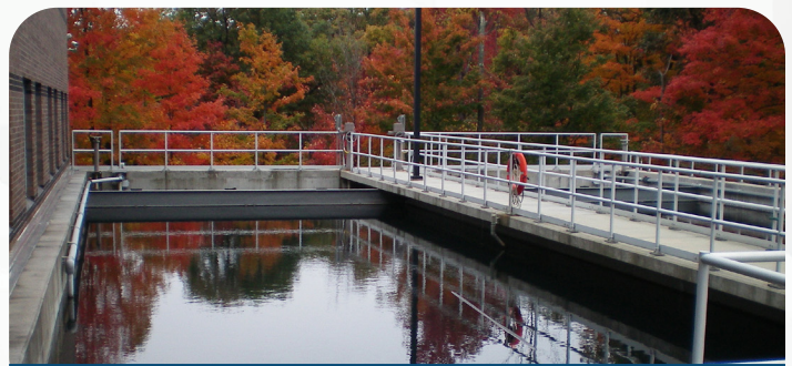
Frostburg Water Treatment Plant
