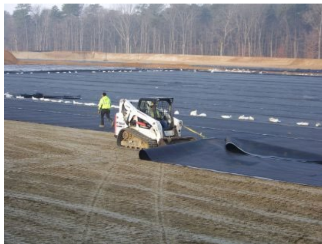
Example of cell construction activities.
