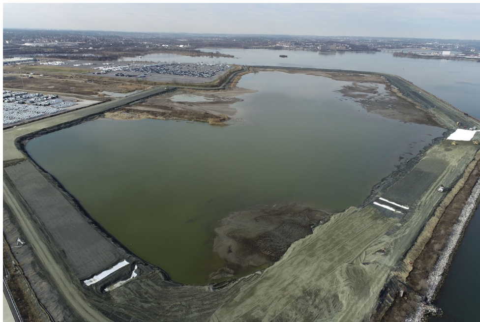
Image 2: Masonville DMCF February 2023 – Base Dike Widening Preparation for +30 Construction
