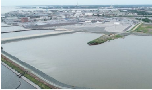
February 2021 Self-Audits at Maryland Department of Transportation Maryland Port Administration Facilities
