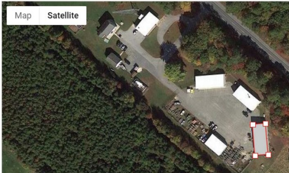
Assateague State Park Building #3 – Carpentry Shop
