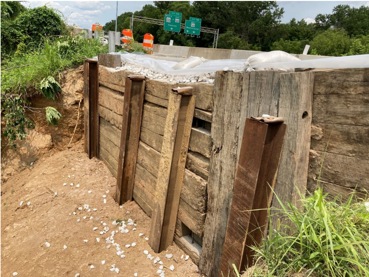
795 Emergency Repair (updated photo and currently active)
