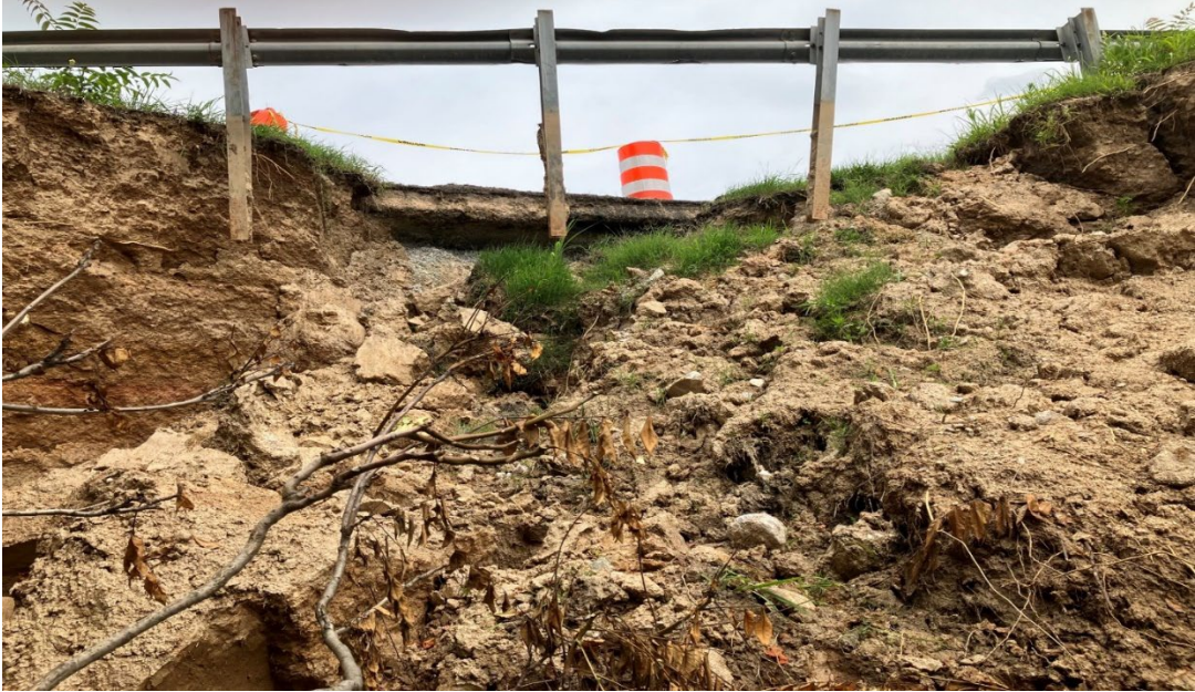
795 Emergency Repair (initial photo)
