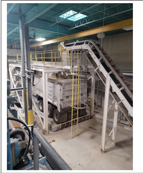
BIOSOLIDS LOADING INTO CONTRACTOR'S PARKED TRAILER AT DORSEY RUN WWTP
