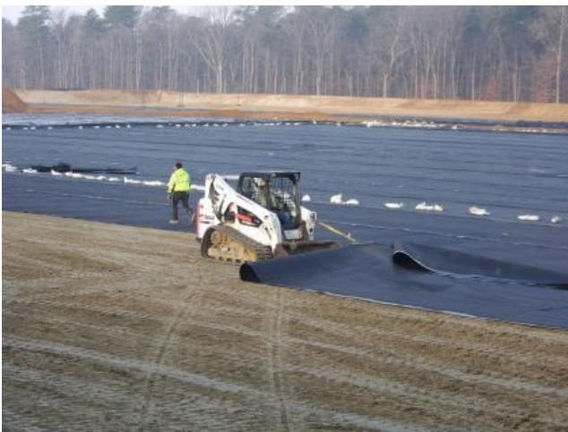
Example of cell construction activities.
