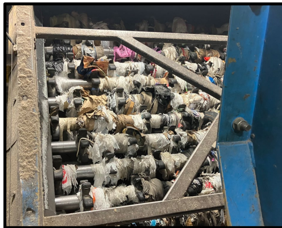
Current screen showcases large plastic buildup
