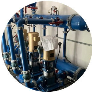
Pictured above, Sandy Point State Park Water Tower, Rocky Gap Membrane Retrofit, and Camp Fretterd Pump Station Upgrade Pictured below, Operations Challenge Team at the Tri-Association Conference
