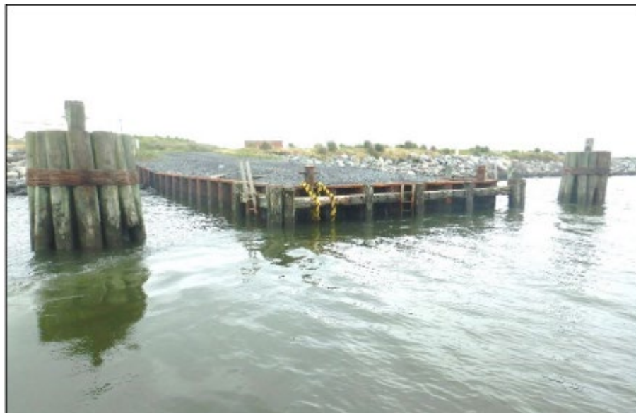
Figure 2. Front View of Poplar Island Fuel Pier Bulkhead and Timber System
