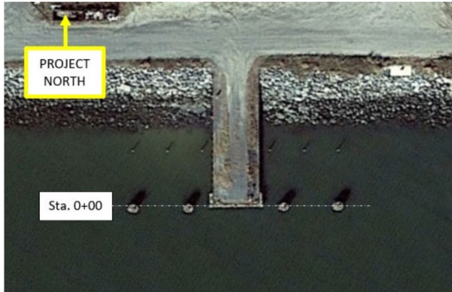
Figure 1. Aerial View of Poplar Island Fuel Pier
