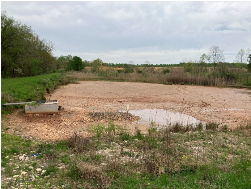
Photo of Barger Tract Pond Sediment buildup
