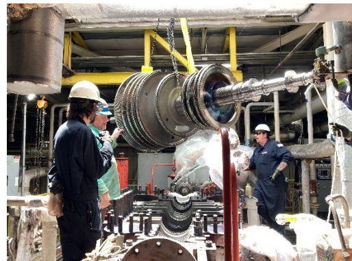
Rotor being installed in steam turbine at ECI.
