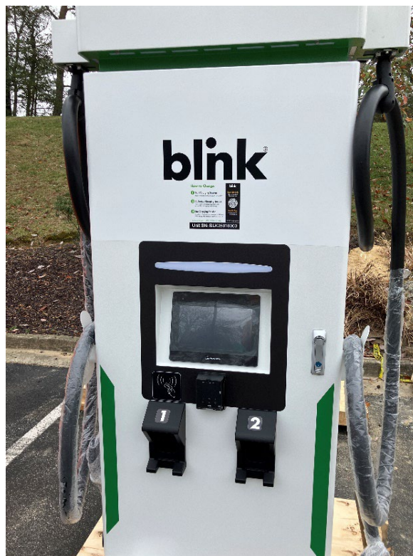
HQ EVSE: Blink Level 2 Charger
