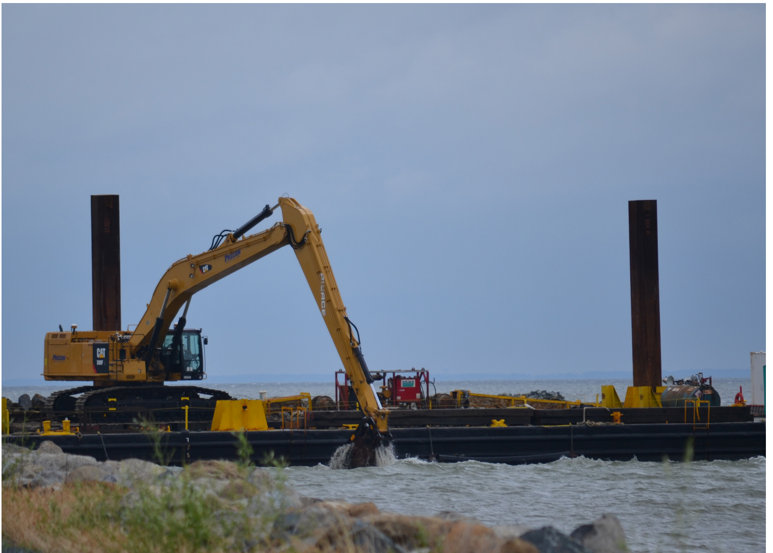
Dredging Equipment at Poplar Island
