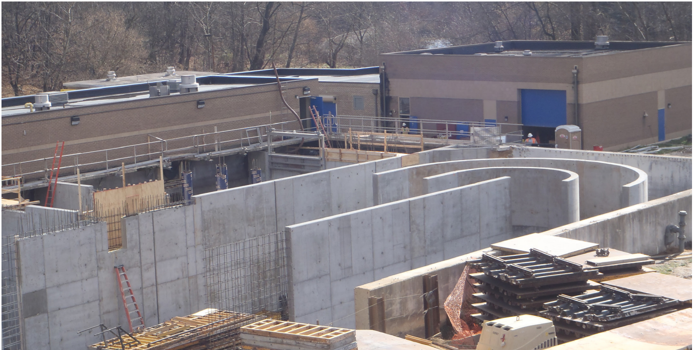
Construction at Freedom Wastewater Treatment Facility
