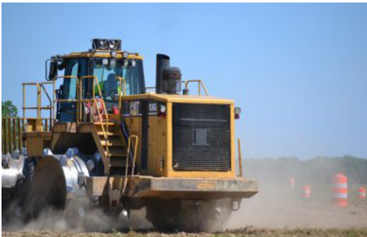
Operations at the Midshore II Regional Landfill
