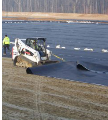
Landfill Cell Construction
