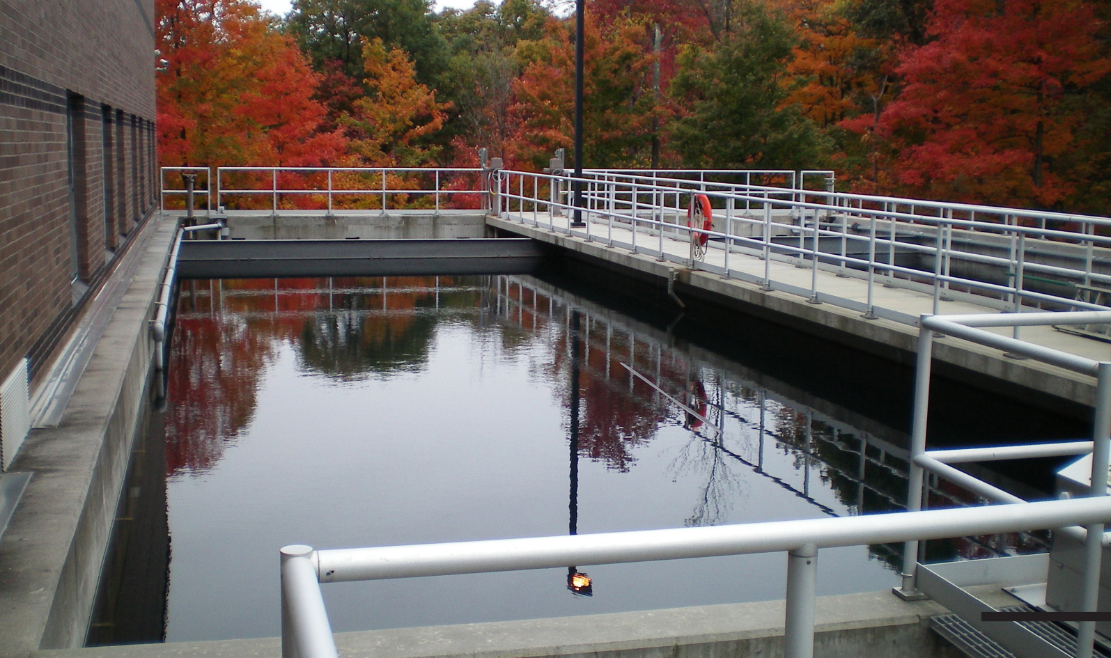
Frostburg Water Treatment Plant
