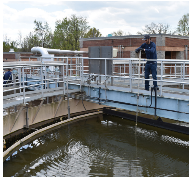
Dorsey Run Wastewater Treatment Facility
