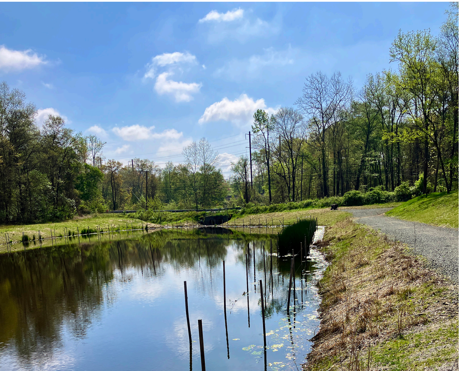
Stormwater Retention Pond
